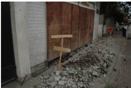
Digging fence foundation.
