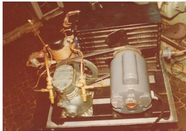
Immediately at left is a standard 3 hp refrigeration condensing unit, which we modified by adding a distillation tank with sight glass, float switches, solenoids (see compete unit on leftmost photo), but most importantly, relay logic circuitry that would automatically draw the oil-refrigerant mixture from the PE chiller's evaporator, then suck off the R-12 refrigerant and pump it back to the chiller's condenser, then pump down the
