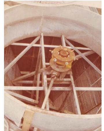
Except for the control panel and CLS semi-hermetic compressor, the water-chiller in the left photo was completely made locally. Center photo was a 15 ton PAC, and again, except for the imported Lau fan and compressor, everything was local. Eventually however, Mr Franco, the Mfg Mgr, developed/manufactured his fan with bad results. His imitation Marley cooling tower, above, was great though.
