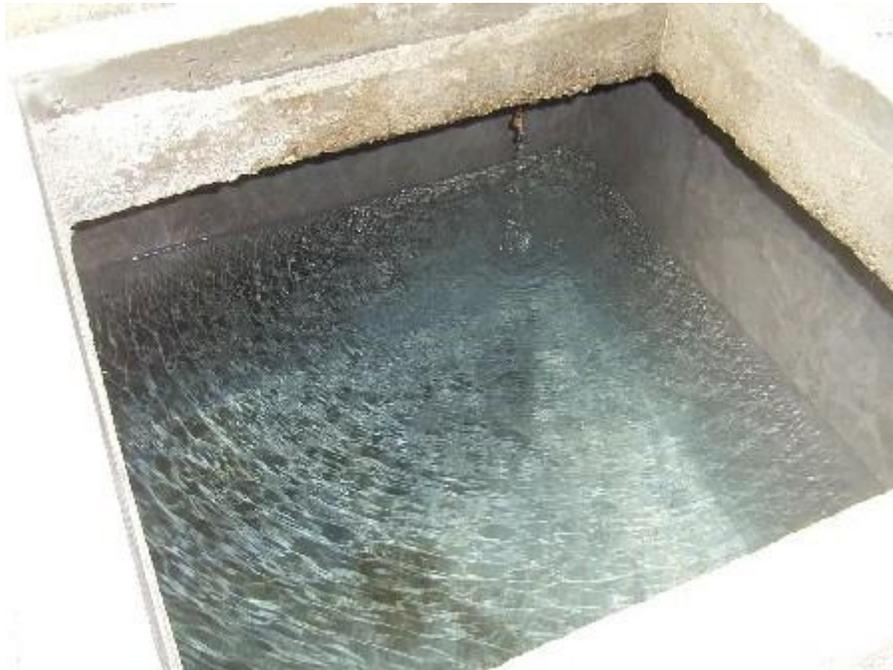
That's fresh spring water passing through a float valve into the cistern. Not visible is a standpipe with foot valve running to a pump.
