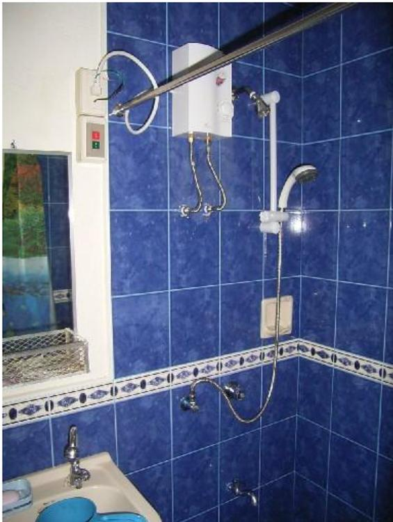
Normally, most homes don't have hot water, but here's the 2nd floor bath with an electric water heater. Note two shower systems. Also note the red/green electric pushbutton station. It is low voltage at 24 volts.
