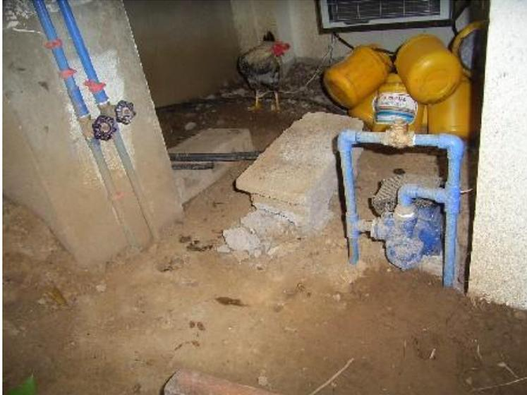
Within the piping system is a 1/2 hp booster pump that I wired up to a control box with an on/off pushbutton station and 10 minute timer, in case one forgets to push the off button. The pump circulates water in a closed loop to boost pressure for showering, and if the pump runs continuously, the street water can't enter to the overhead tank. The pump cannot suck from the main street line because it is against the law. The chicken in the background was a delicious meal later that evening.
