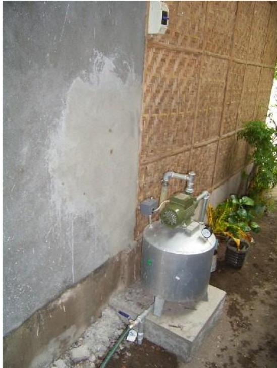
The \$32 contraption is a combination 1/2 hp Italian pump with locally made GI pressure tank, a US-make pressure switch, and valving. This allows for strong running water needed especially in the outdoor shower after a dip in the sea. Notice the juxtaposition of a concrete wall (the indoor bathroom) and the woven-bamboo-slat wall (the kitchen).
