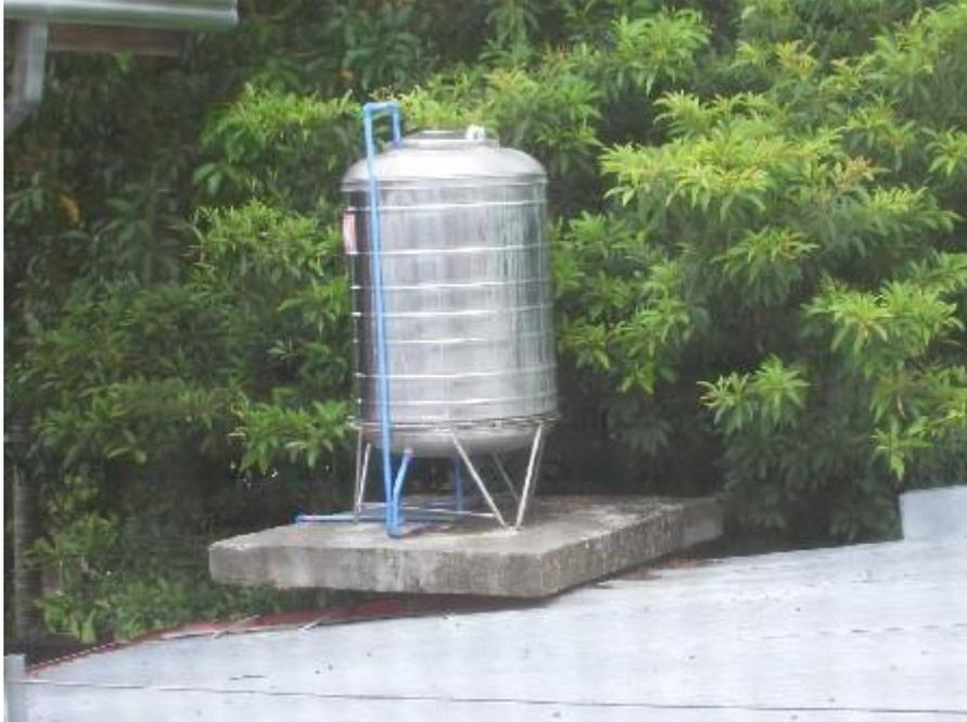
The SS overhead water tank at our house in the town proper is at a lower level than the 2nd floor bathroom. Street water pressure is quite strong during early morning hours, and float valve on inlet pipe prevents water from overflowing.
