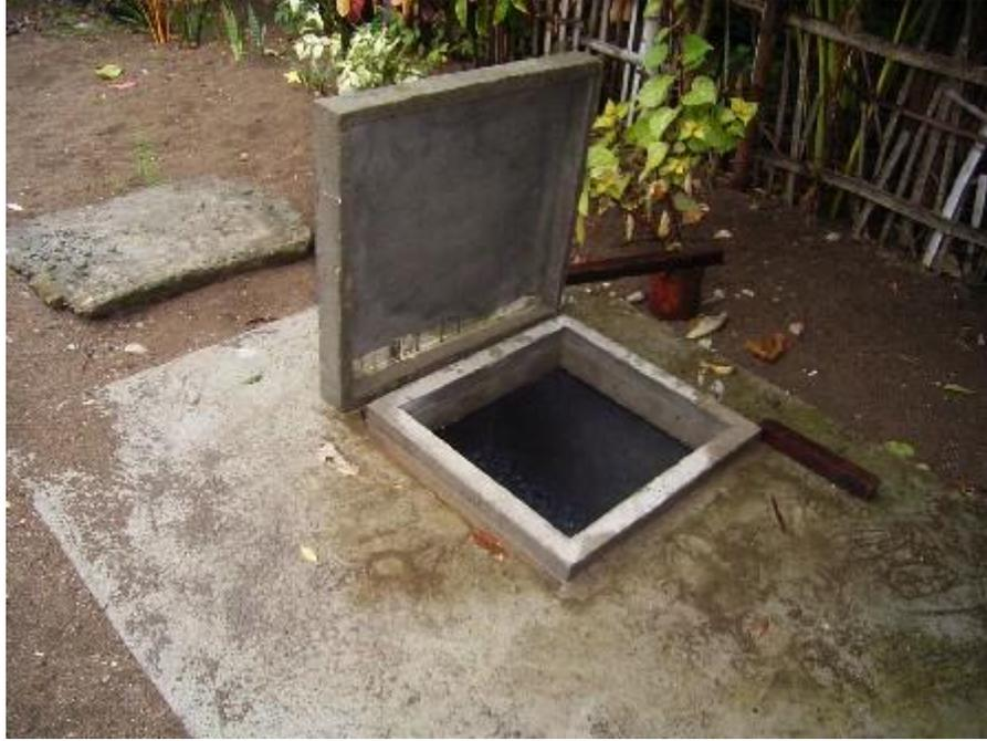
The situation at the beach house a few miles away from town is quite different. Water pressure is so low it wouldn't be able to go to an overhead tank. The water is sourced directly from a spring at the nearby mountains and runs down by gravity. Seems like a half inch pipe services about a dozen huts. So, we built an underground cistern in the sand, holding 3 cubic meters.
