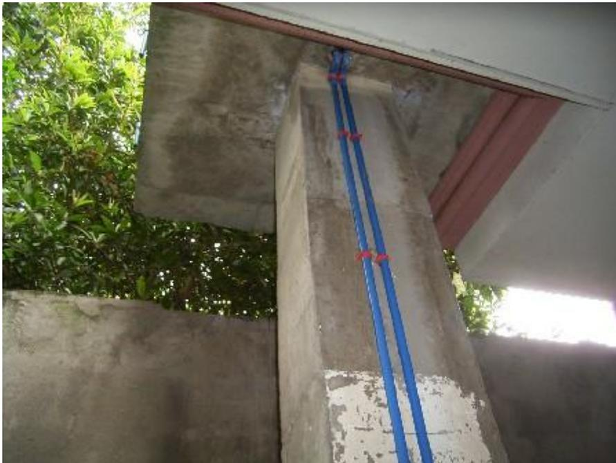
Inlet and outlet PVC pipes run up to the overhead tank, with float, check and isolation valves to automatically store water in tank and prevent it from running back to the street main line when mains supply pressure is low.
