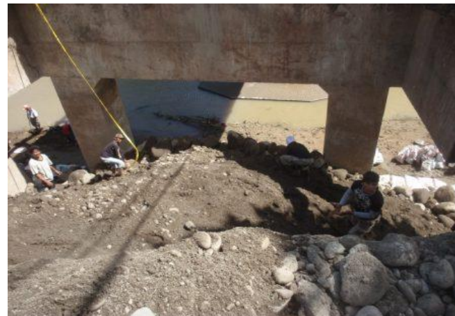
Left, middle & right views of eroded side of bridge, Dec 19. Dept of Public Works personnel working to build back retaining wall and embankment.
