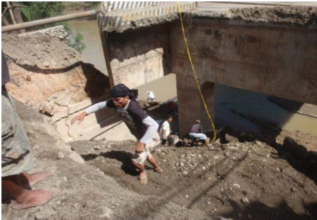
Left, middle & right views of eroded side of bridge, Dec 19. Dept of Public Works personnel working to build back retaining wall and embankment.
