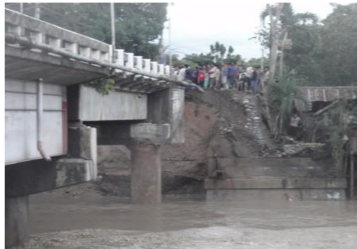
Telephoto shot of washed out bridge approach, north side
