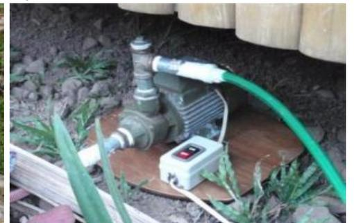
But the 18 rows of veggie plots with similar perforated hoses had to have a pressure source: an economical small 1/3 hp pump, with valving to feed 1 or 2 rows at a time, squirting water for 10 minutes for each set. However, with the pump put off, the same effect can be achieved over a number of hours of slow dripping by gravity. It's just a matter of fine tuning the system.
