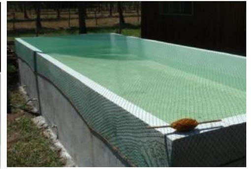
The float valve that shuts off when full.
