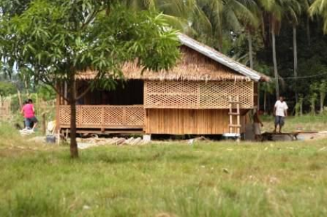
Almost completed rest house.
