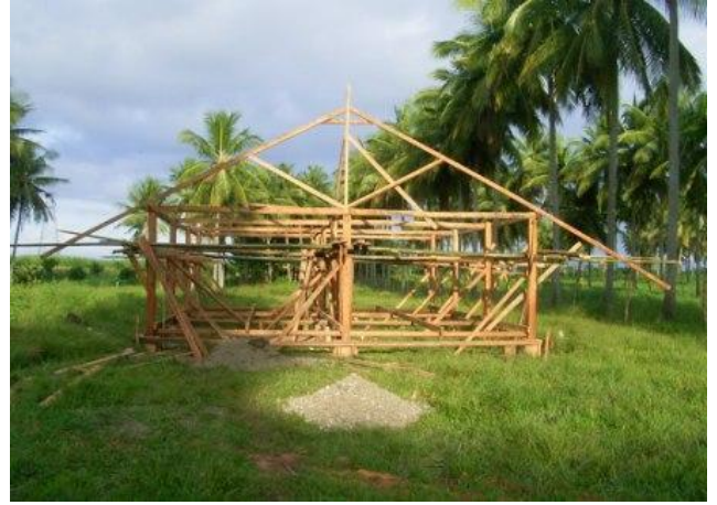
Day 6 of work. I find the local term for the roof A-frame, visual: "sala-gunting", meaning scissors.
