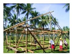
No need for gu-od footings, then with the coco floor joists, and bamboo roof framing, it takes shape.
