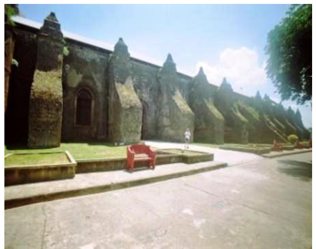
Paoay right side wall and line of buttresses.
