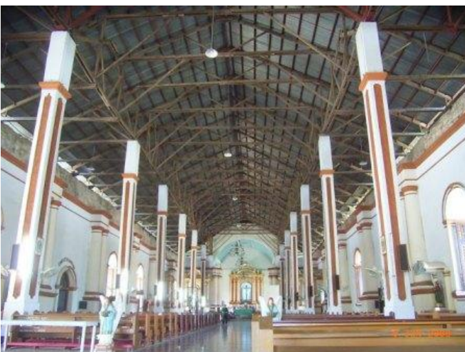
Inside Paoay church, new roof, mainly held up by pillars.
