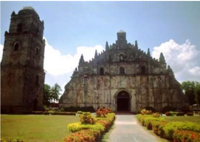
Paoay church, with preserved façade and bell tower. Church cornerstone laid 1704; bell tower 1793.
