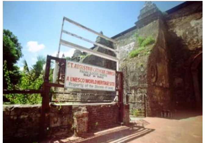
Sign indicating it is a World Heritage Site, with flying buttress reinforcing left side wall.
